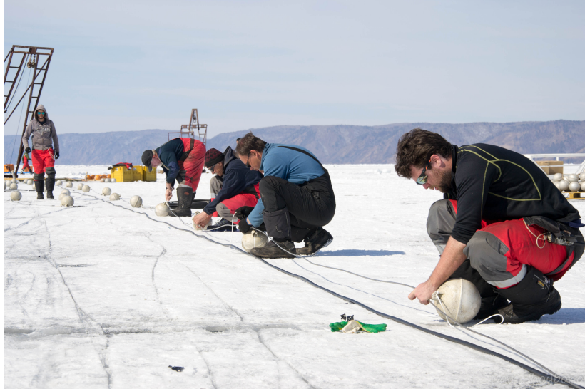
Figure 7: Picture of the installation works on the surface of the frozen lake. The author of the thesis is first from right.
